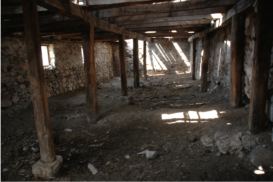
FIGURE 13.4 Monastery in Ch'arek'tar partially re-adapted, photos: 'Monument Watch'
