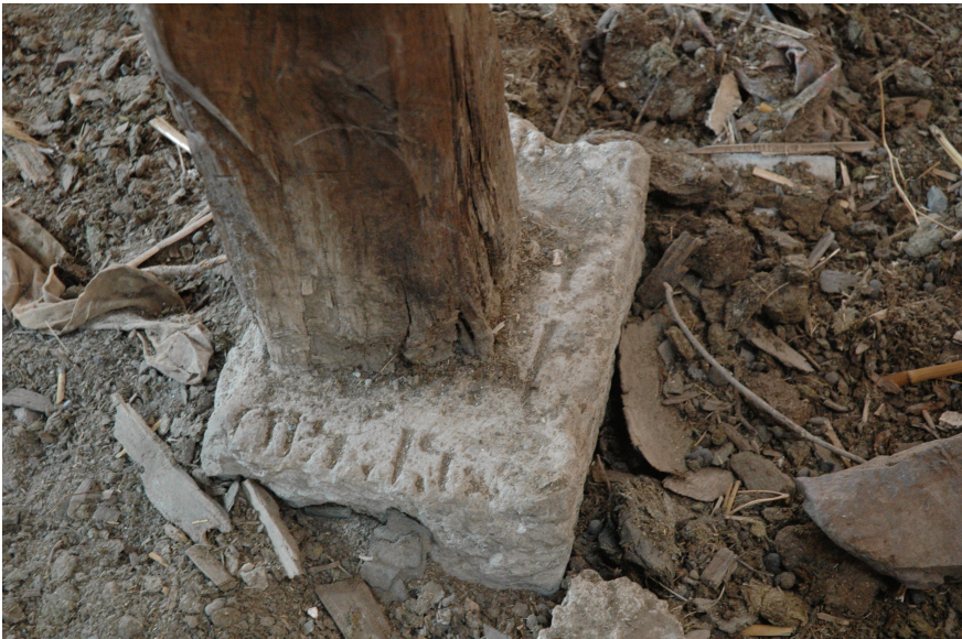
FIGURE 13.5 Monastery in Ch'arek'tar partially re-adapted, photos: 'Monument Watch'
