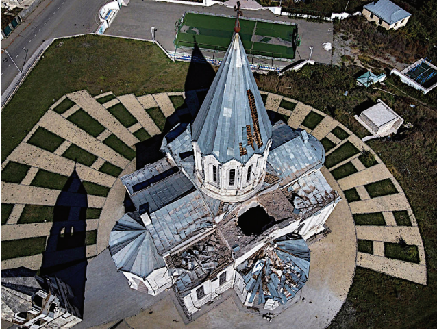
FIGURE 13.8 Cathedral of the Holy Saviour (Łazanch'ets'ots'), Shushi, photos: 'Monument Watch'
